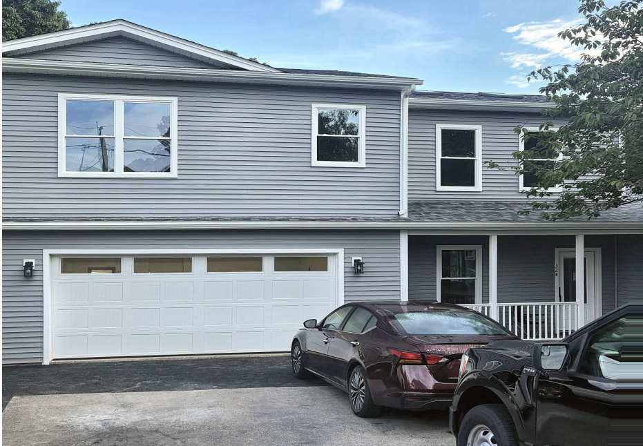
COMPLETED — THE FULL FRONT ELEVATION. THE ADU OCCUPIES THE SECOND STORY OVER THE EXISTING TWO-CAR GARAGE; THE NEW MUDROOM AND COVERED ENTRY TIE IT TO THE ORIGINAL 1966 RANCH.
