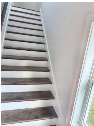
OAK-TREAD INTERIOR STAIR
